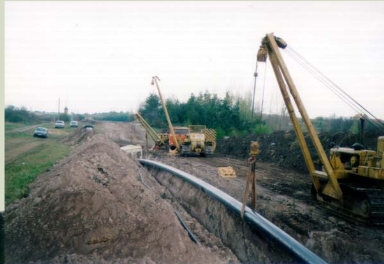
raw material pipeline Rostock-Boehlen under construction
