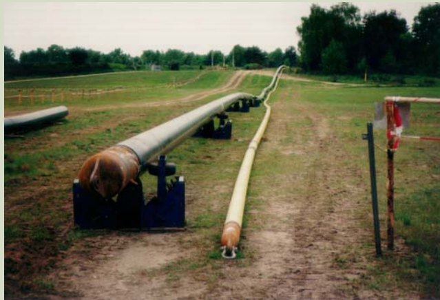
pipe and cable protecting casing prepared for underpass crossing canal Mueritz-Elde
